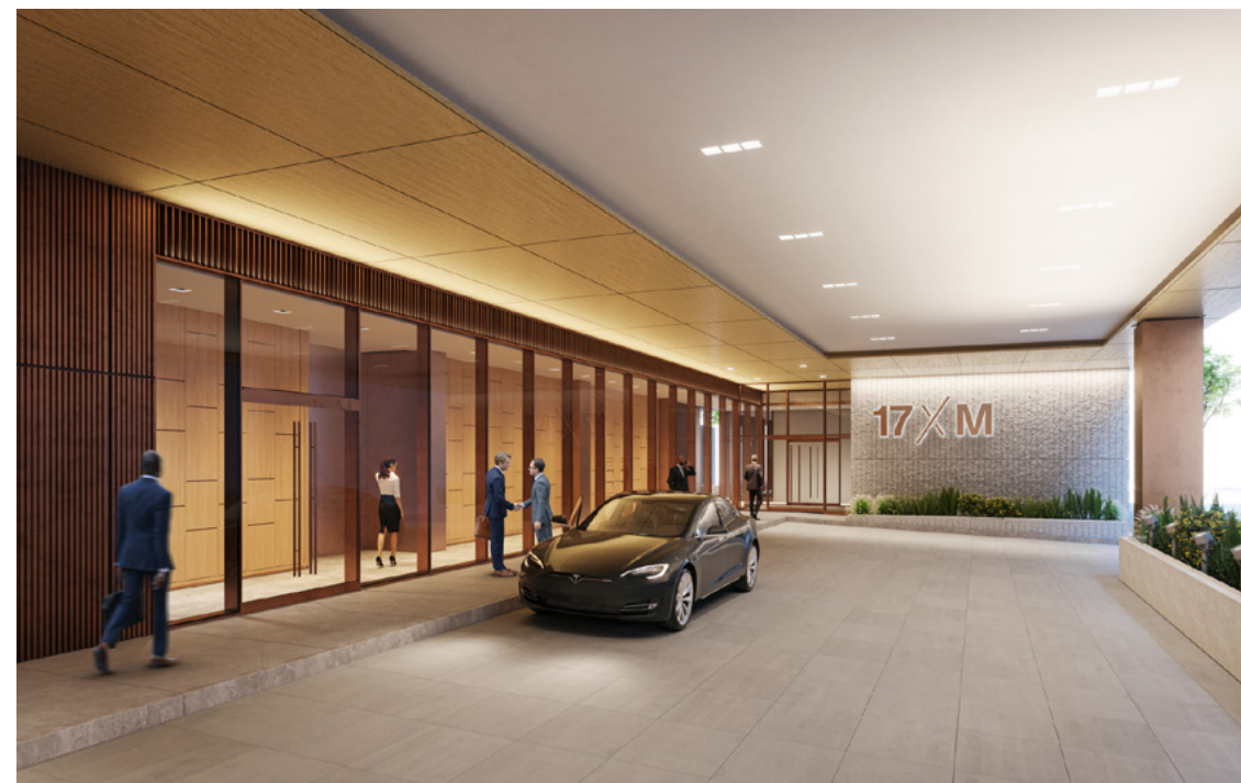
Through smart access technologies, credentialed visitors can enter through 17xM's rear, porte-cochere entrance.
