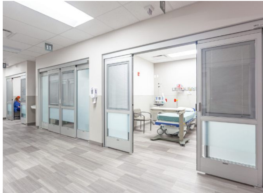
Figure 1: Suites within a hospital facility are used to comply with NFPA 101 requirements while keeping patient comfort and care as a top priority. Courtesy: Jacia Phillips, Henderson Engineers
