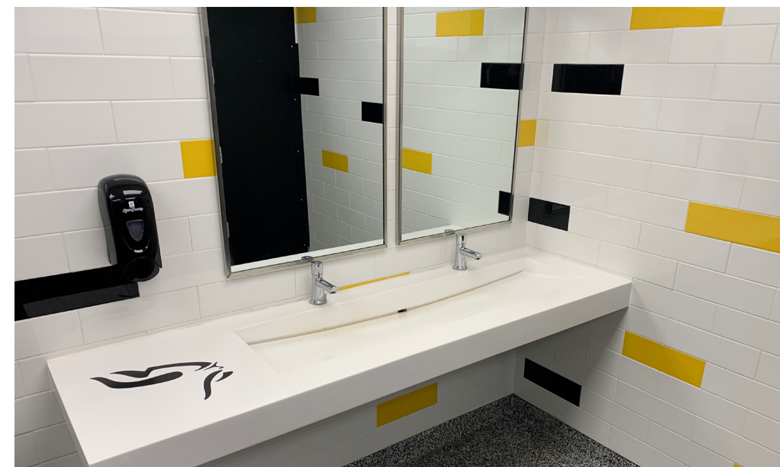
Tri-County Schools in Howard City, Michigan wanted a quality faucet with uniformity, clean look and low maintenance. Tri County preferred the 3500 Series metering faucet. The 3500 Series offers a metered cycle with a timed automatic shut-off, adjustable anytime between two to 25 seconds after turning on to conserve water.
