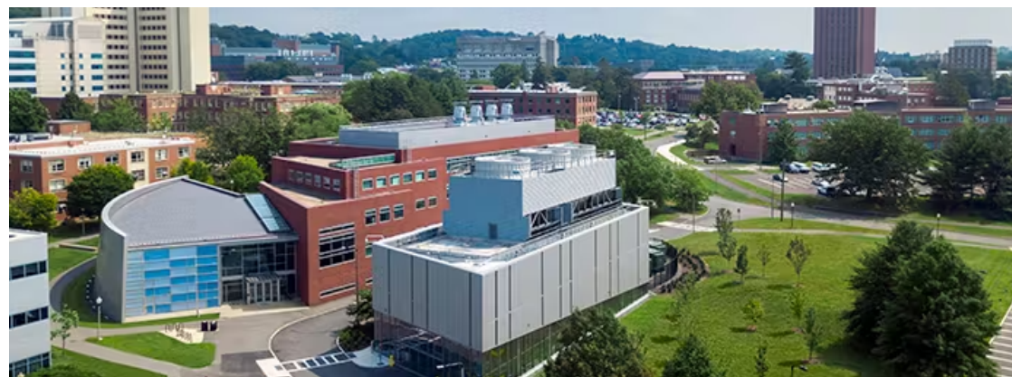
University of Massachusetts Amherst North Chiller Plant
