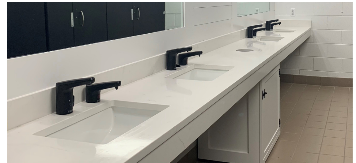
Northpointe Christian Schools in Grand Rapids, Michigan wanted an upscale look for their new restroom renovation. They selected the E-Tronic 80 touchless faucet and soap dispenser in matte black because it is both easy to maintain, as well as stylish for a modern look. The E-Tronic 80 has easy to access above-deck electronics, integrated ASSE 1070 certified scald protection, optional user adjustable temperature control and is easy to adjust and monitor with the CF Connect app. It is the ultimate in restroom hygiene, convenience, and reliability.
