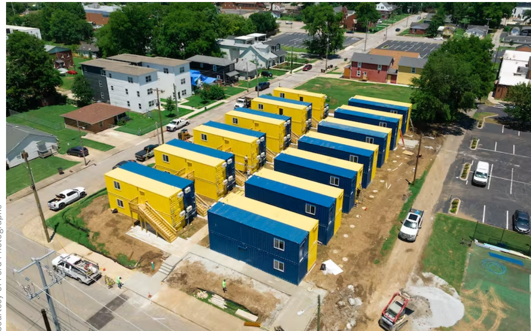
Fisk University used shipping containers to address a housing shortage on campus. Each container has one efficiency apartment for two students.
