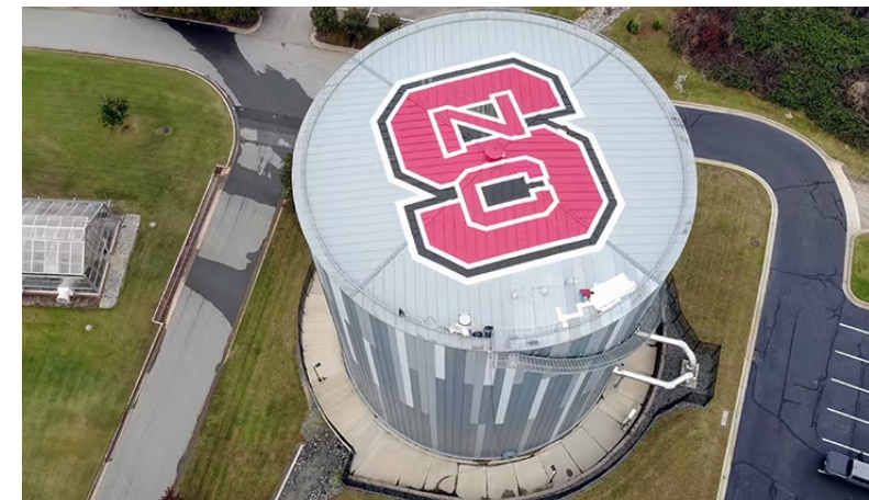
A thermal storage energy tank on the Centennial Campus of North Carolina State University in Raleigh.
