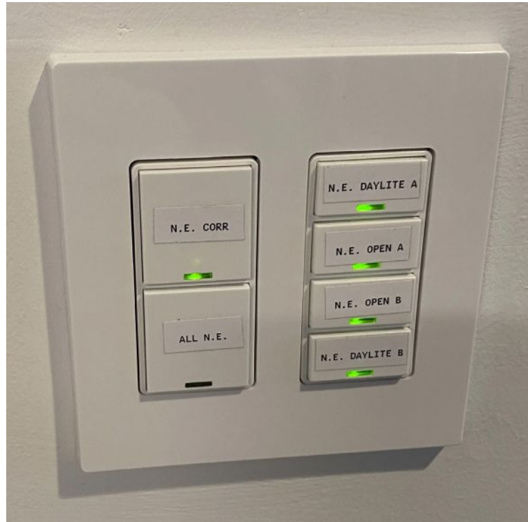
Figure 4: Pictures of lighting control stations with and without labeling. Courtesy: McGuire Engineers
