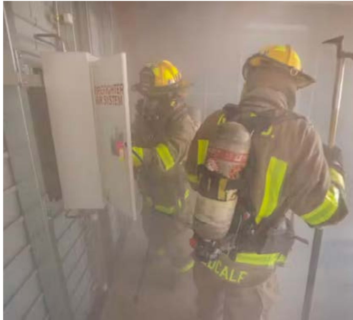
Firefighter air replenishment systems (FARS) stations are designed to refill a self-contained breathing apparatus (SCBA) in up to two minutes, while the firefighter remains protected under full respiration.
