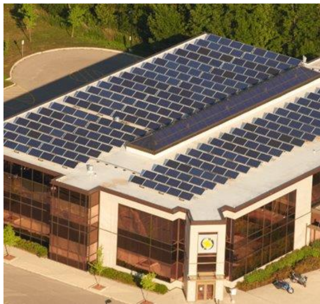
Solar PV array contributes to a cleaner electrical grid
