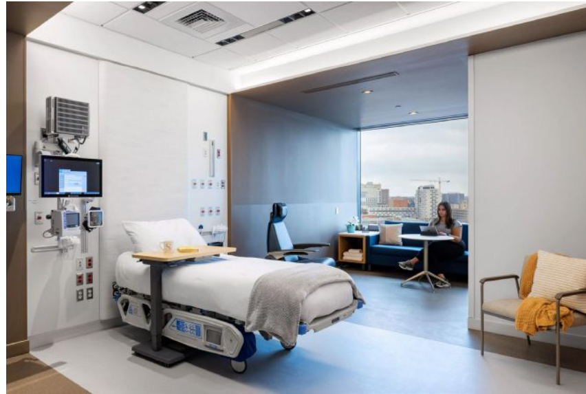
Figure 2: Patient room with lighting keypads on the headwall and in the family zone. Ambient, uplight, charting and family zone on. Shades are up for daylighting and views toward the city. Courtesy: HDR, Dan Schwalm PennFIRST
