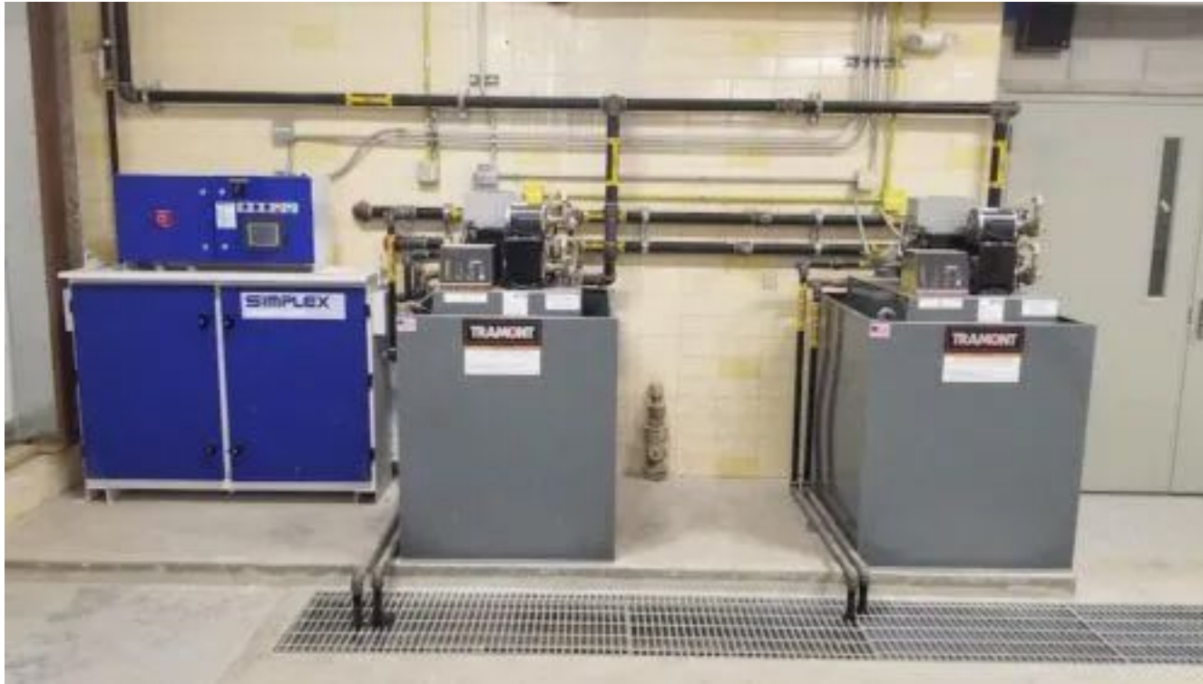
Figure 2: Image of fuel polishing system installed on an existing fuel oil system for improved reliability of relocated generators. Courtesy: IMEG Corp.
