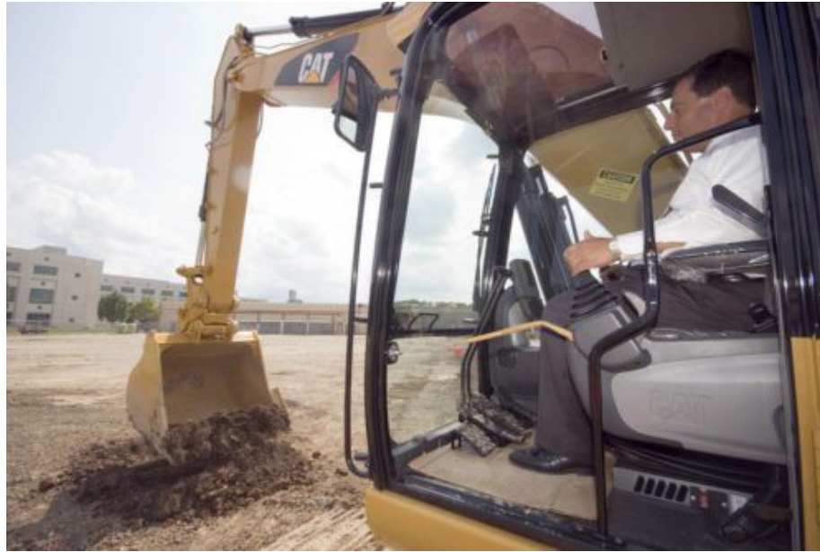
Construction worker breaks ground on sloped site. Courtesy: IPS
