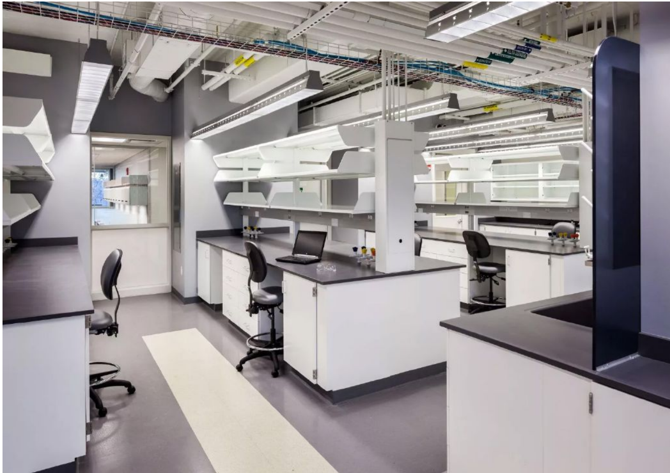
Figure 1: This shows an example of laboratory lighting that is aligned with the edge of bench eliminating the need for undershelf task lights and luminaires located in the circulation corridor. Courtesy: HDR
