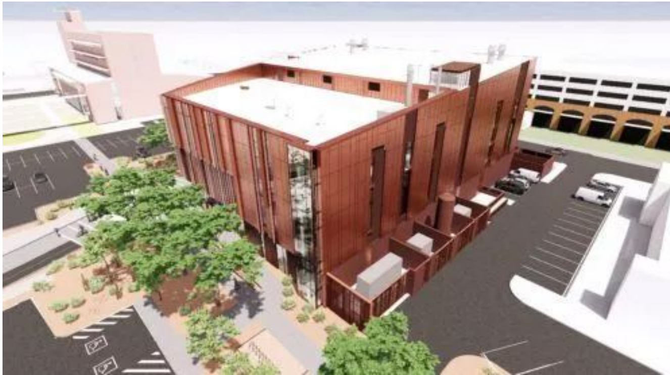
Figure 1: Perspective rendering of utility yard including generator, medium-voltage transformer and medium-voltage switch, located behind an architectural screen wall, emphasizing the visual cohesion between the utility space and the building exterior, at the Applied Research Building in Tucson, Arizona. Courtesy: Ryan Haines, SmithGroup
