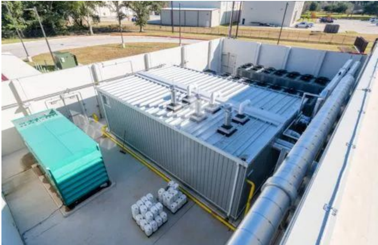
Figure 3: A generator appears in a chiller yard with a utility transformer in the distance, located in Texas. Courtesy: Wade Griffith, SmithGroup
