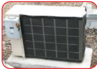
AIR COOLED CONDENSER INTAKE FILTER
