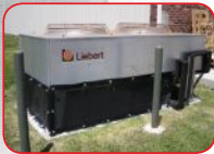
DRY COOLER INTAKE FILTERS
