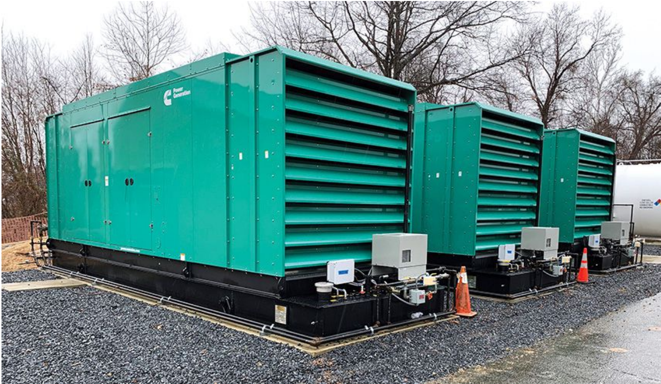
Figure 5: Installation of three 750-kilowatt diesel generators in weatherproof enclosures at MedStar St. Mary's Hospital installed as part of the emergency power upgrades project. Courtesy: CMI General Contractors
