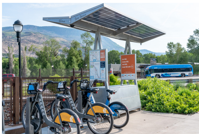
A solar canopy powers an electric bikeshare charging station in Basalt, Colorado. This innovative application of a solar canopy was developed by WE-cycle in partnership with Skyhook Solar and PBSC Urban Solutions. Source: Craig Turpin, Rising Sun Photography
