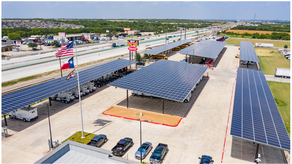
Parking canopies installed in San Antonio as part of the Big Sun Community Solar Program protect vehicles from hail damage, direct sun, and excess heat. Source: Big Sun Solar, 2020
