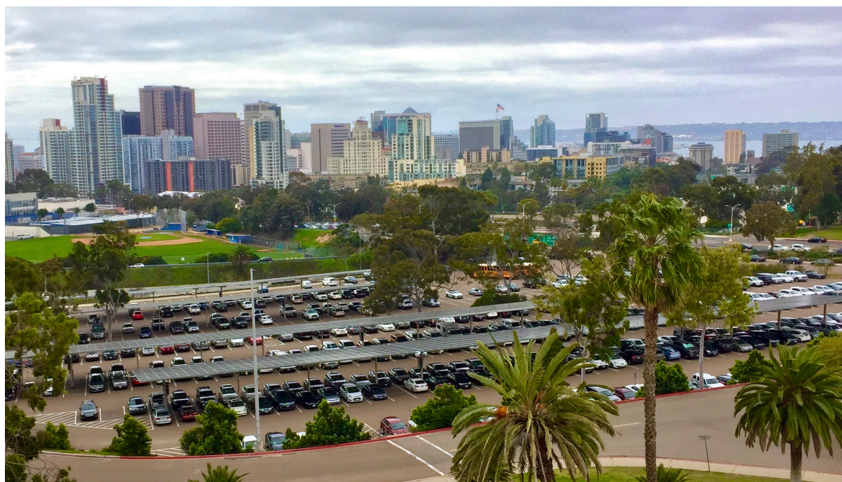
Though not community solar, the City of San Diego's 983 kW parking canopy in Balboa Park is the largest and cheapest project on a per-kWh basis of the 14 distinct rooftop and parking canopy solar projects installed by the city. Source: City of San Diego, 2020
