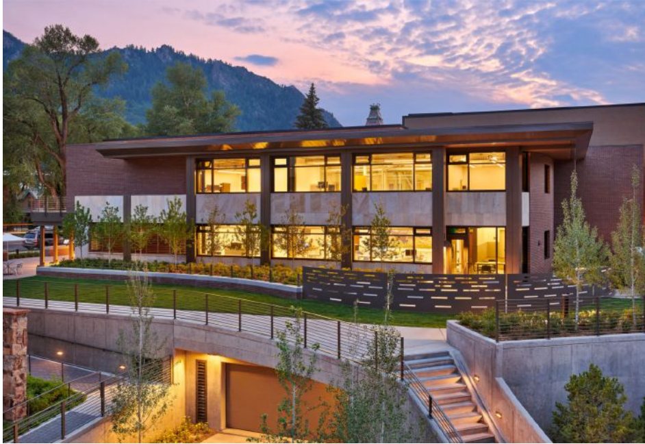
Figure 2: Automated operable windows at the WELL certified Aspen (Colo.) Police Department not only reduce energy consumption by providing free cooling they also significantly increase the supply of outdoor air directly to the occupants, further promoting a connection to the outdoors. Courtesy: Dallas & Harris Photography, IMEG Corp.
