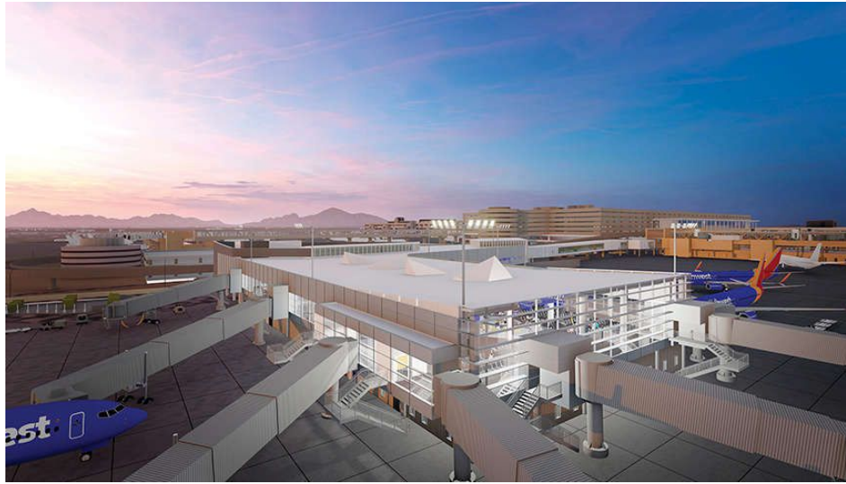
Figure 5: New concourse expansion at Phoenix Sky Harbor International Airport will provide additional gates for airlines to use. Courtesy: SmithGroup
