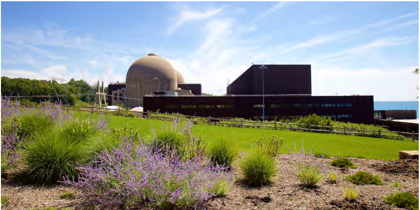
The Donald C. Cook Nuclear Power Plant, on the shores of Lake Michigan, has upgraded its cooling systems to mitigate rising water temperatures from the lake.
