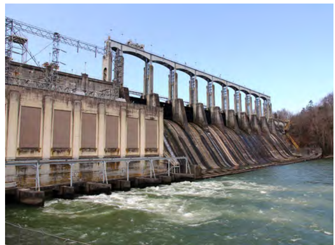
AEP's 75 MW Claylor Lake Hydroelectric Facility in Virginia.
