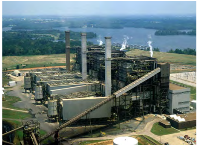
Welsh Plant will cease coal operations in 2028.
