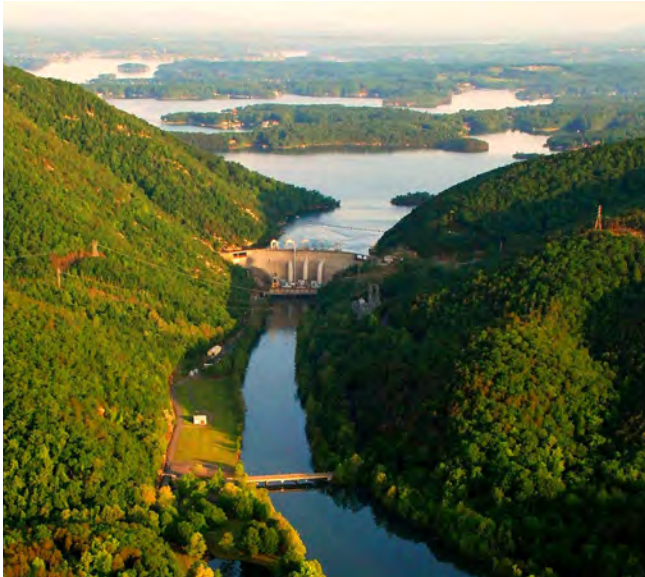
Appalachian Power's Smith Mountain Pumped Storage Facility in Virginia can provide up to 586 MW of electricity.
