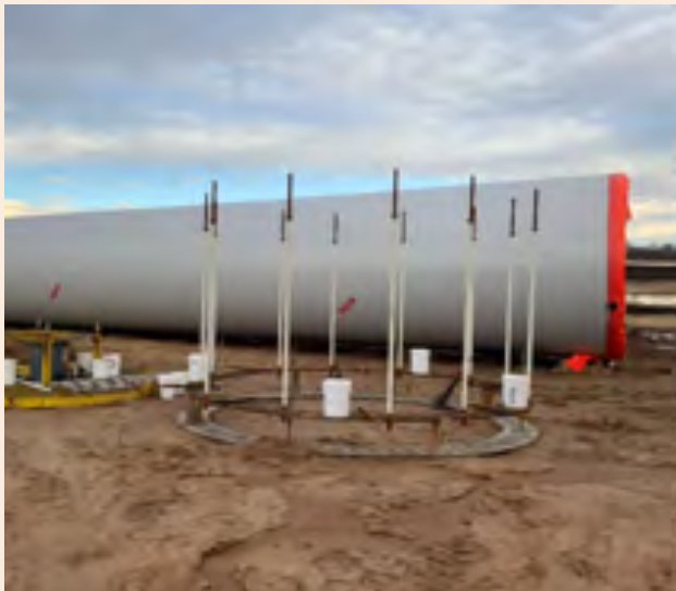
Construction is underway on the 1,485 MW North Central Wind.
