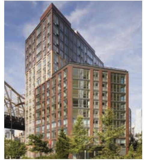
Like many buildings of the era and typology, extensive glazing is common. Photo Credit: Steven Winter Associates
