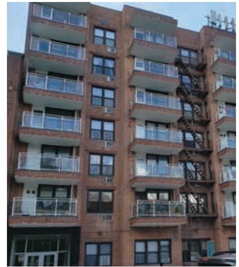
The study building includes common features like low performance glazing systems and balconies. Photo credit: Steven Winter Associates
