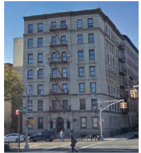
Like many buildings of this era and typology, the building features punched windows and a largely opaque facade. Photo credit: Steven Winter Associates
