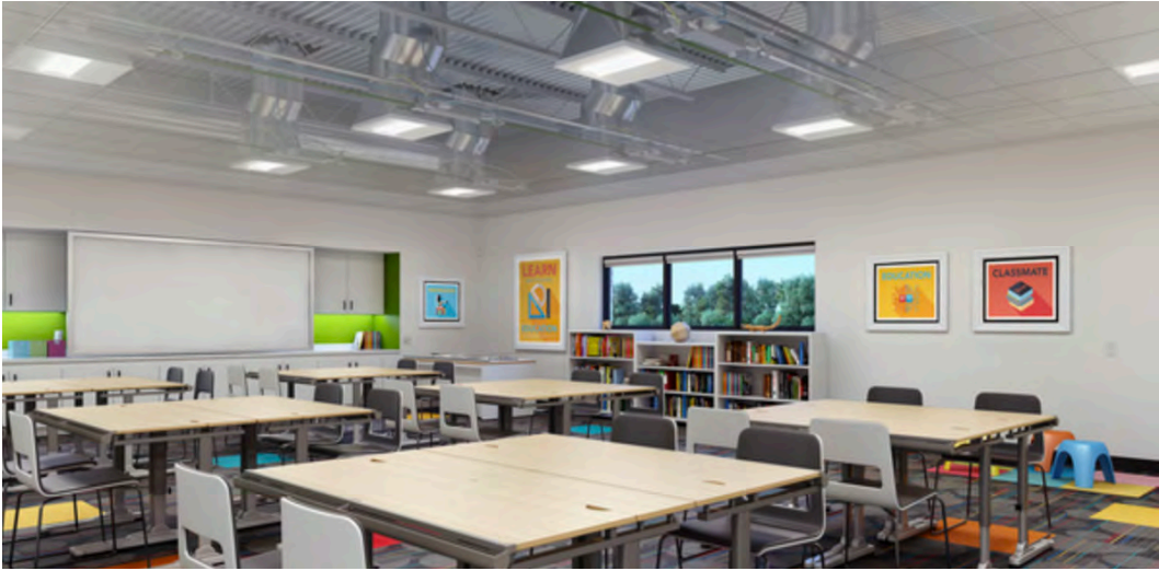
LightFlex LED with tunable white lighting in a classroom. Credit: Sunoptics
