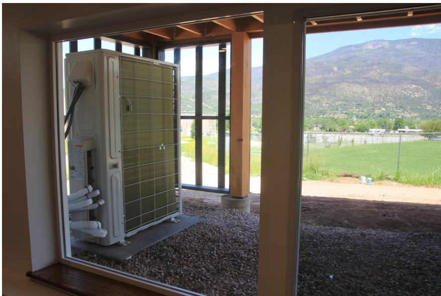
Figure 4.2.13. Air source heat pump (Best, 2020).
