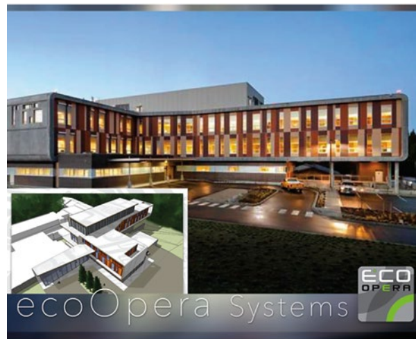
Figure 3-8 Eco Opera Systems at Vancouver Coastal Health Authority
