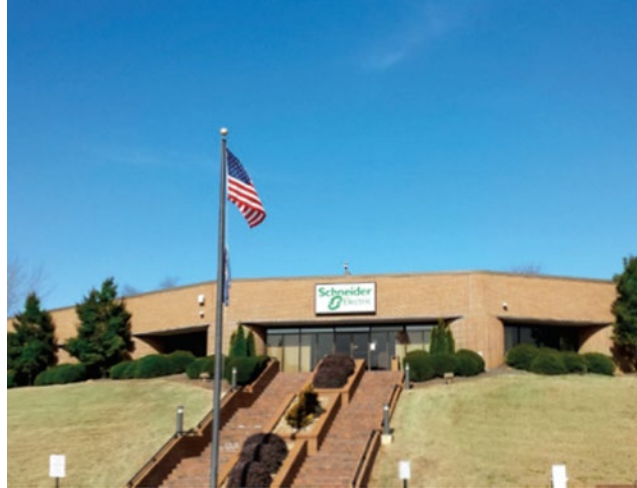
Figure 3-16 Schneider Electric’s Seneca Manufacturing Facility
