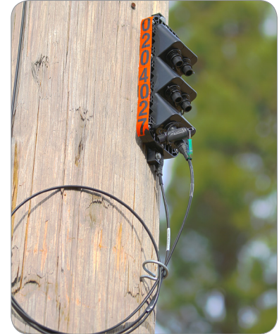
Figure 5 — Multipoint terminal with hardened drop connectors installed.
