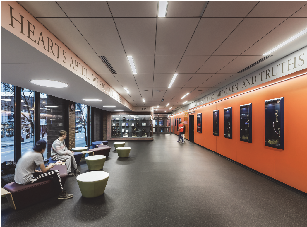
Figure 5-29 (EL10) Example of asymmetric versus symmetric luminaire layouts. Photo courtesy Ballogg Photo.com, Nagle Hartray Architecture, IMEG Corp. Lighting Design & Engineering
