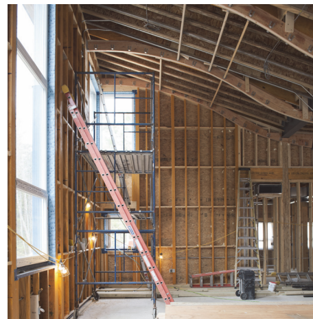
Construction of meeting room.
