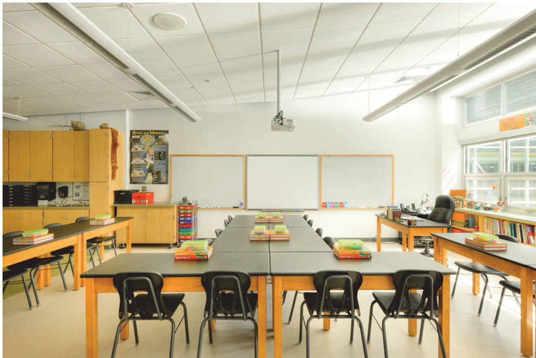
Figure 5-24 (DL15) Light redirection in a classroom. Photo © Sam Kittner/Kittner.com, provided courtesy of LightLouver LLC
