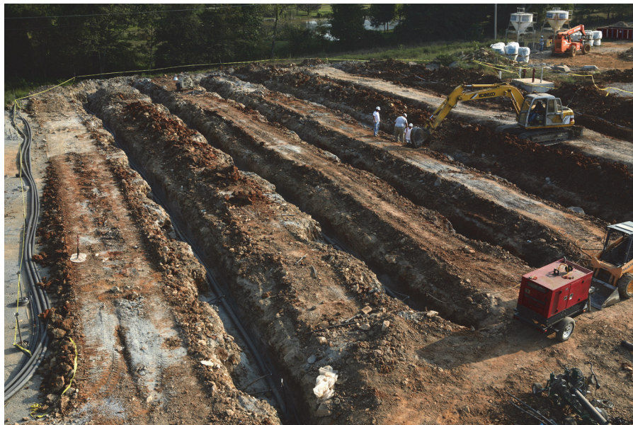
Figure 5-45 (HV11) Geothermal field horizontal trenches. Photo reprinted with permission of CMTA
