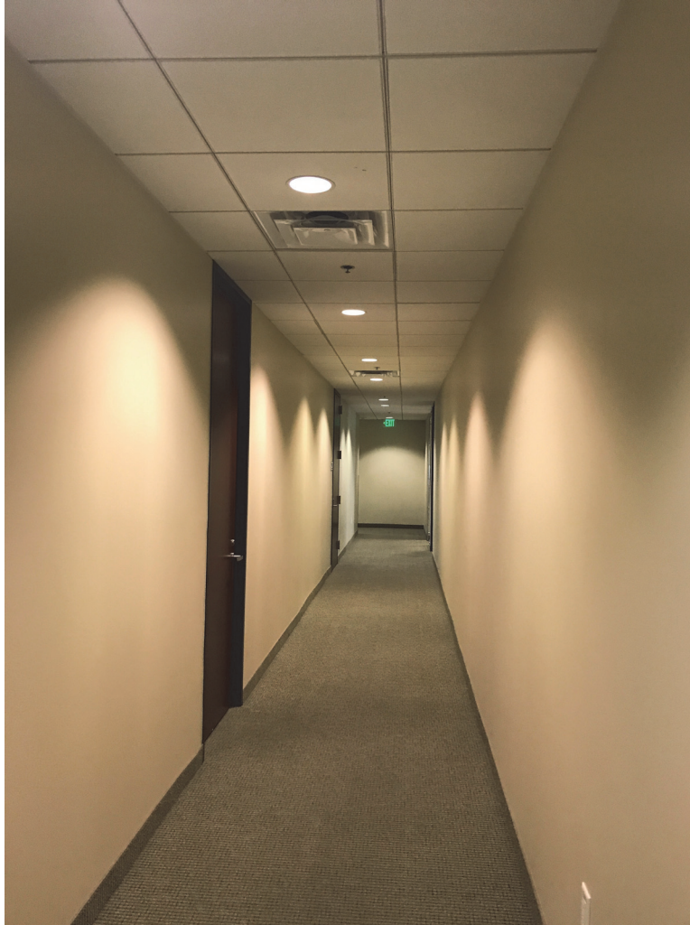
Figure 5-28 (EL9) Example of scalloping patterns and dark ceilings. Photo reproduced with permission by Shanna Olson
